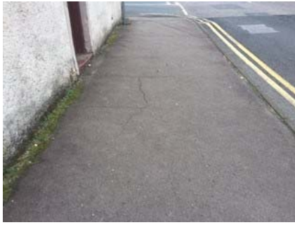
Footway—adjacent to the carriageway
